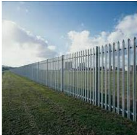
Plate 3-15. Standard palisade fencing
