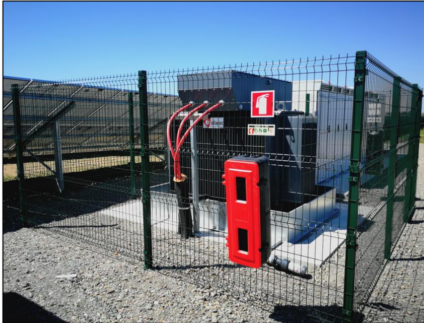
Plate 3-14. Typical transformer compound fencing
