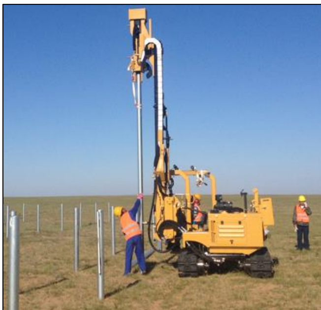
Plate 3-18. Ramming of module mounting structures.
